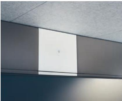
Presence detector, temperature sensor and CO<sub>2</sub> sensor are used for fully automatic control of lighting and ventilation
