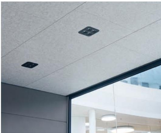
The PET felt panels in the ceiling and the fully insulated technical wall significantly improve the reverberation time of this “room-in-room” system.
